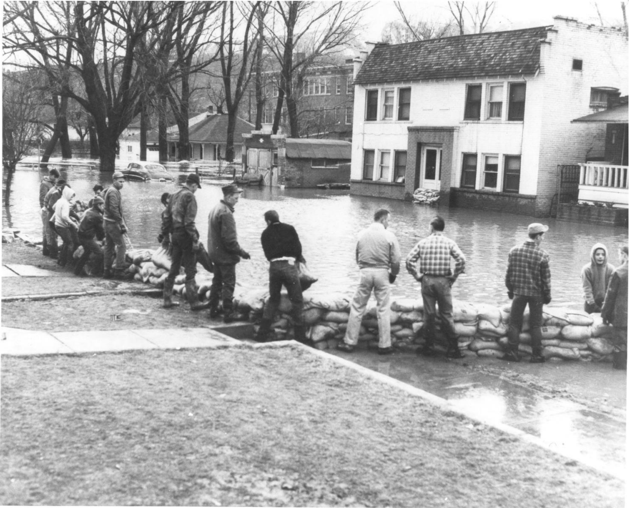
Figure 12 – Sandbag Levee Construction 1962 (City of Pocatello, 2015)
