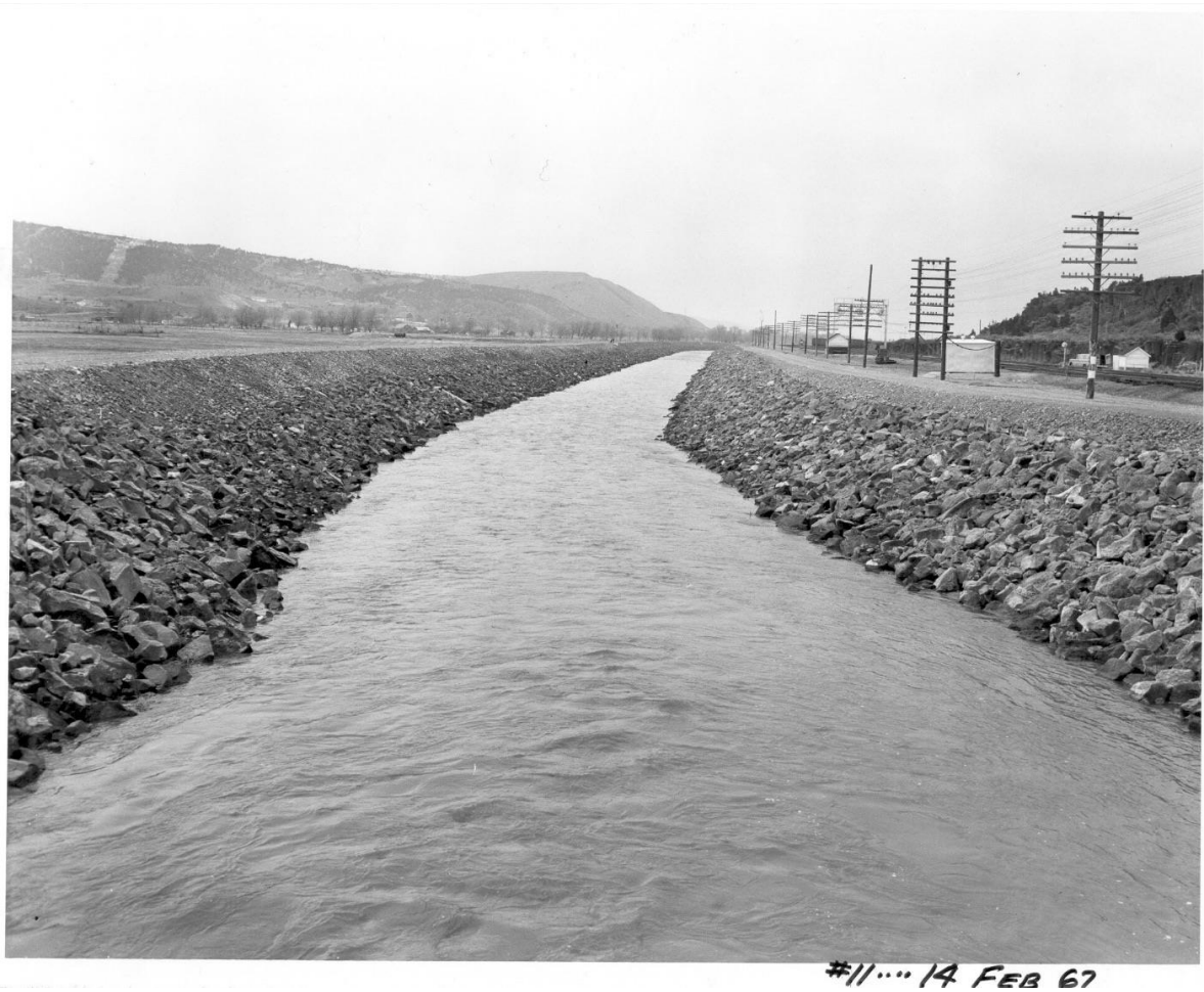
Figure 14 – Levee Channel Modification 1967 (City of Pocatello, 2015)
