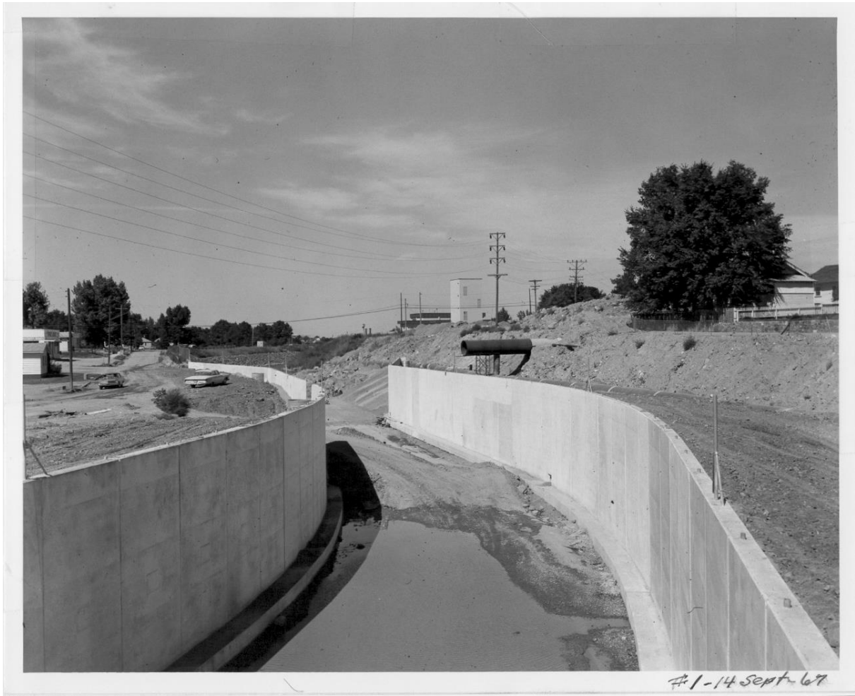
Figure 13 – Concrete Channel Modification 1967 (City of Pocatello, 2015)
