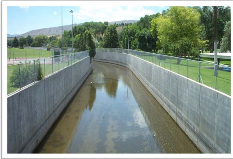
Figure 2 - Concrete Channel Section
